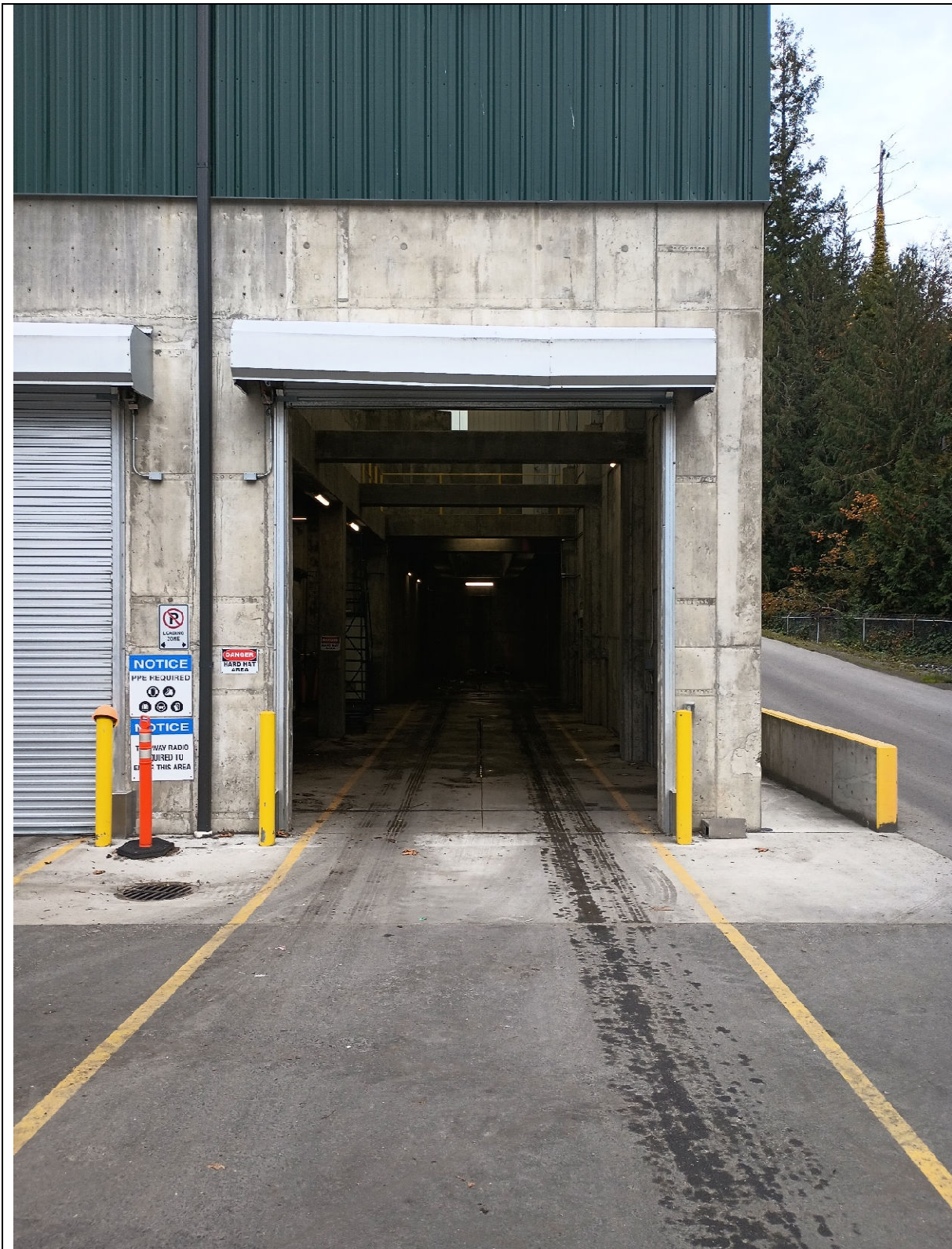
MWS LOADING AREA ENTRY DOOR
