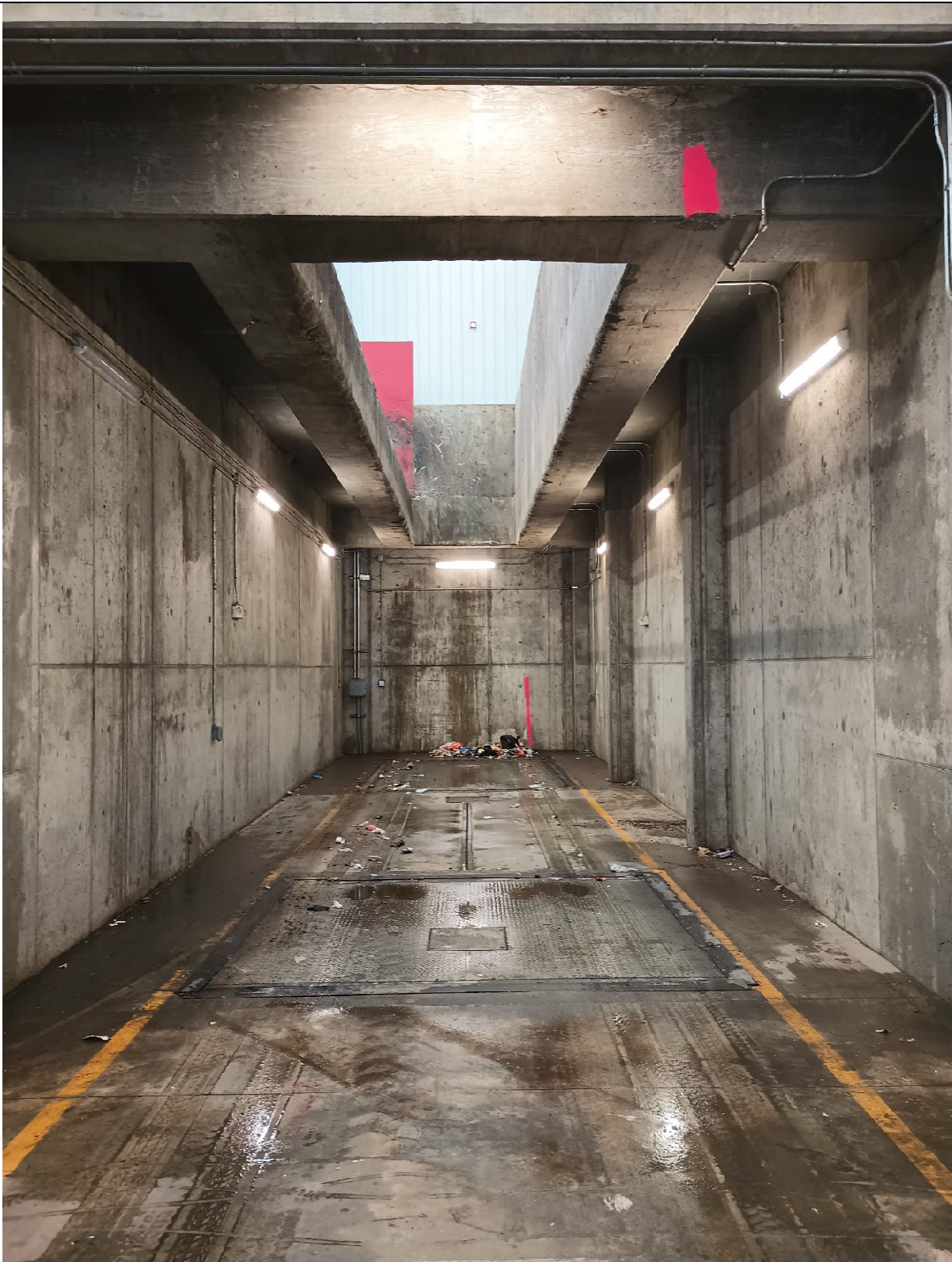
MSW LOADING AREA AND SCALE PLATFORM
