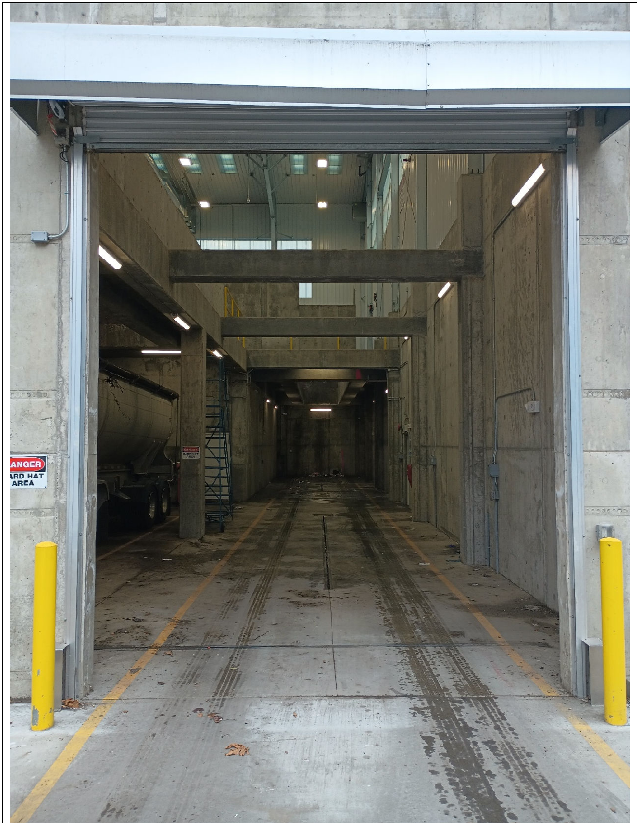
MWS LOADING AREA
