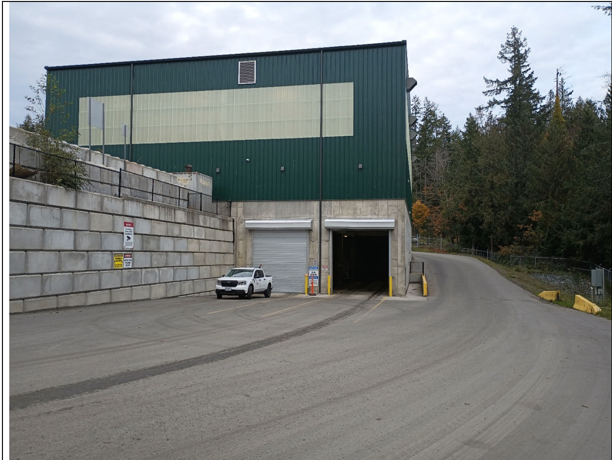
TRANSFER STATION AND ACCESS ROAD
