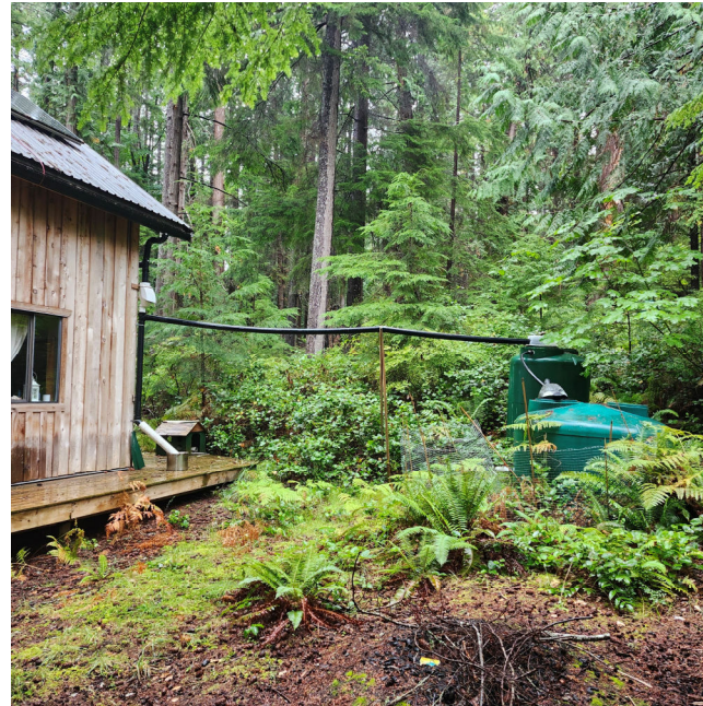
Rainwater catchment system on east Savary Island
