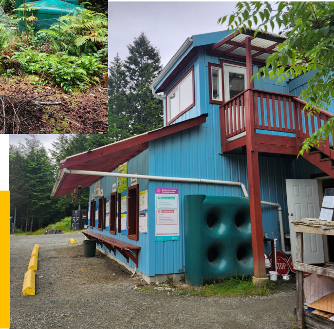
Rainwater catchment system at Cortes Island Recycle Depot
