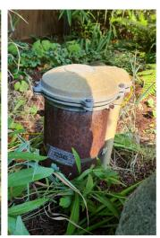
**Drilled wells** for household use are usually 6 inches in diameter with a steel casing and are usually deeper than dug or driven wells
