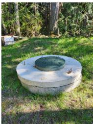
**Excavated (dug) wells** are typically larger in diameter and shallow, with sides made of cement or wood cribbing
